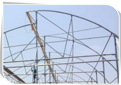
Poly House Structure
