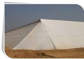
Wire Rope Shed Net House
